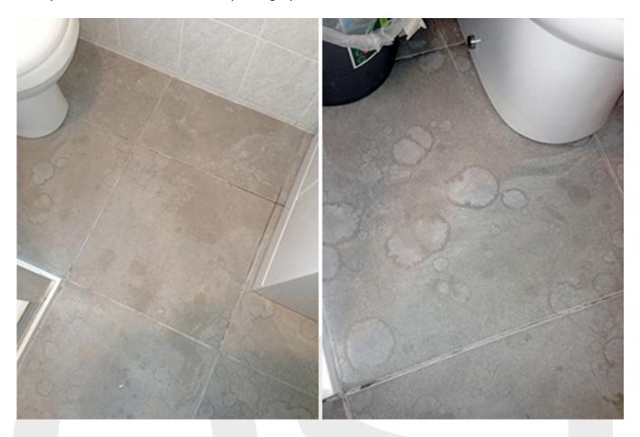
This dried surface residue ordinarily appears when it has completely set and more often because the tiles have become wet through cleaning, thus highlighting cement residues, grout stain, efflorescence and other similar deposits randomly across the top of the tiles as they become dry.
